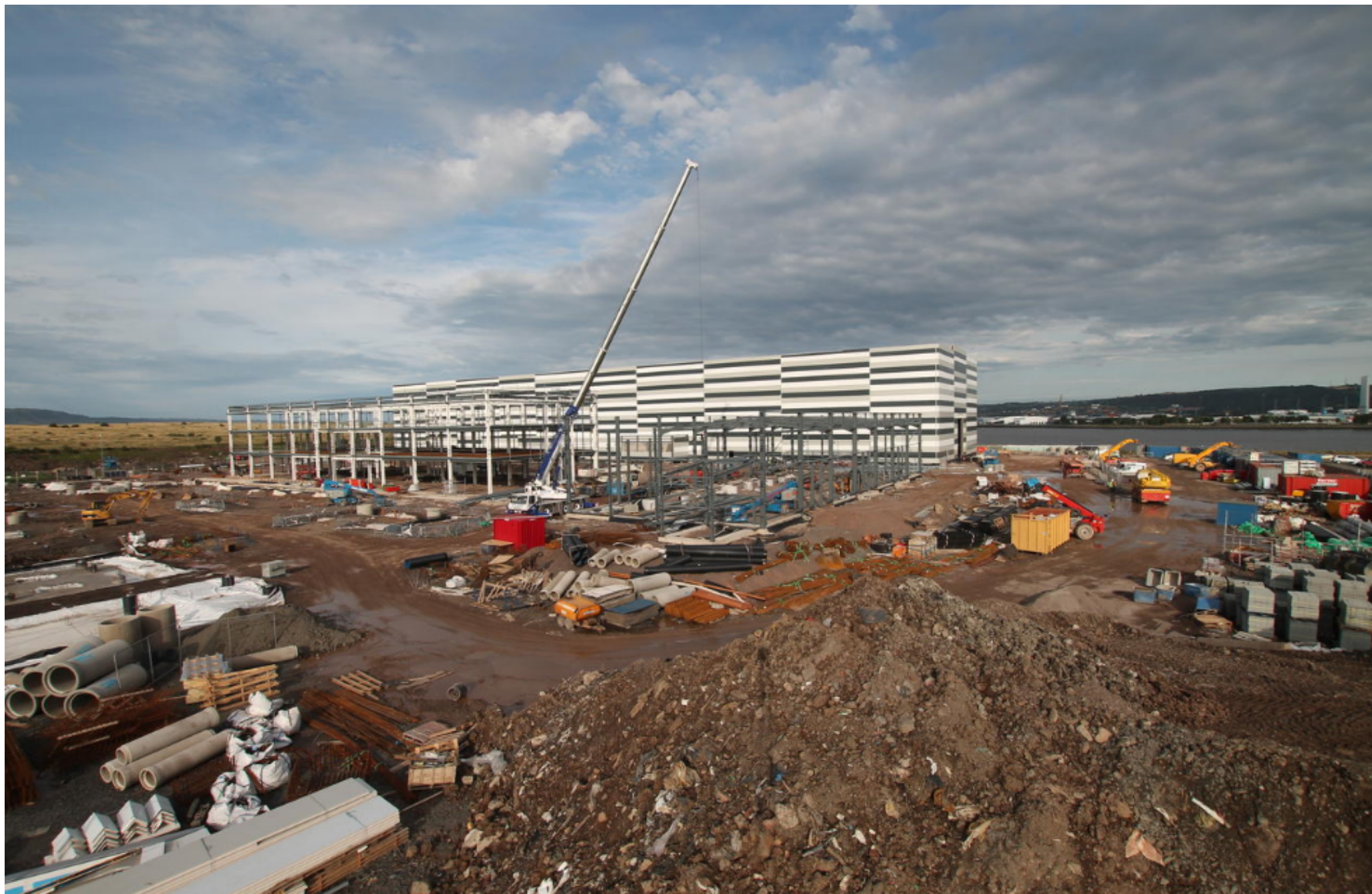
North Foreshore – UNDERWAY
